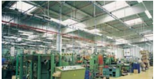
Assembly workshop Transair Ø 63 and Ø 25
